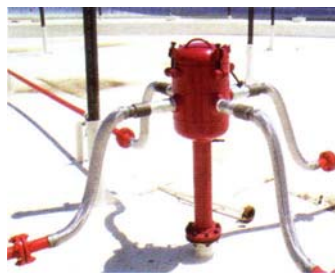
The Mesa Foam Delivery System (FDS) is an efficient method to extinguish rim fires on floating roof storage tanks
