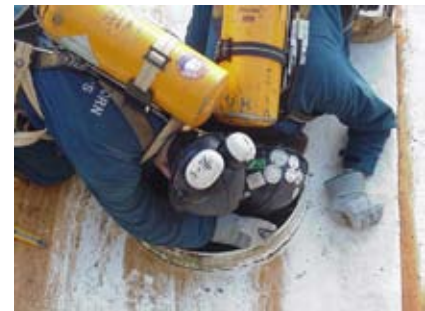
Pontoon Liner is inserted into floating roof.
