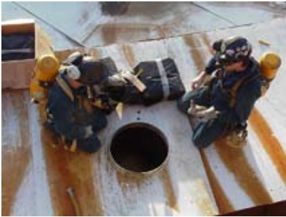
Service technicians prepare to insert Pontoon Liner into roof.
