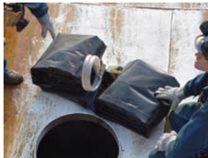
Pontoon Liner is kept in folded position and inserted into roof.
