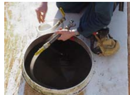
Air inlet is made ready for air connection.
