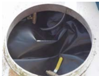
Pontoon Liner is inflated within the floating roof.
