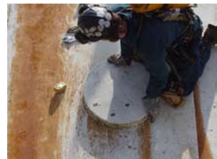
Cover is replaced.
