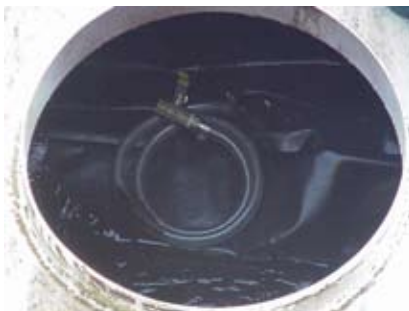
Air inlet on Pontoon Liner is facing upwards for access.
