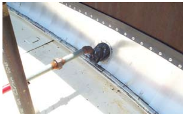
Below Seal Application showing seal boot
