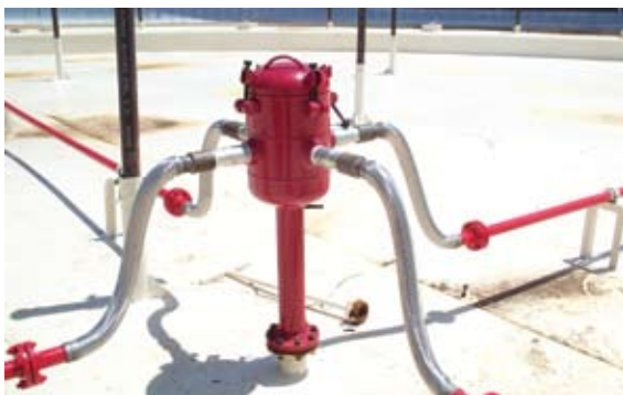
Foam manifold and stainless flex connectors
